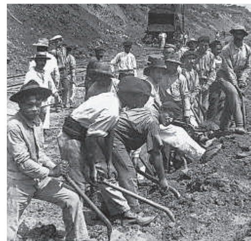
▲ Workers digging the Panama Canal faced hazardous landslides and death from disease.
